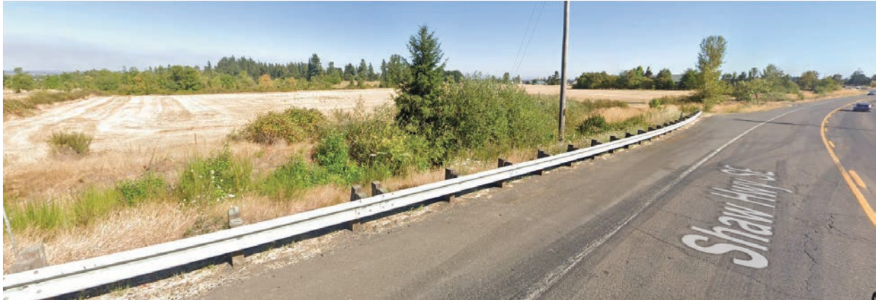
Figure 2: Street View looking east from Shaw Hwy
